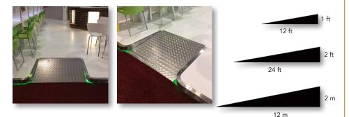
**In addition** to beveled slopes and ramp requirements, further suggestions to clearly highlight a change in floor levels are shown below.
